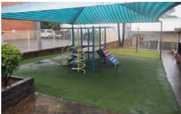
The playground area was in need of upgrade
